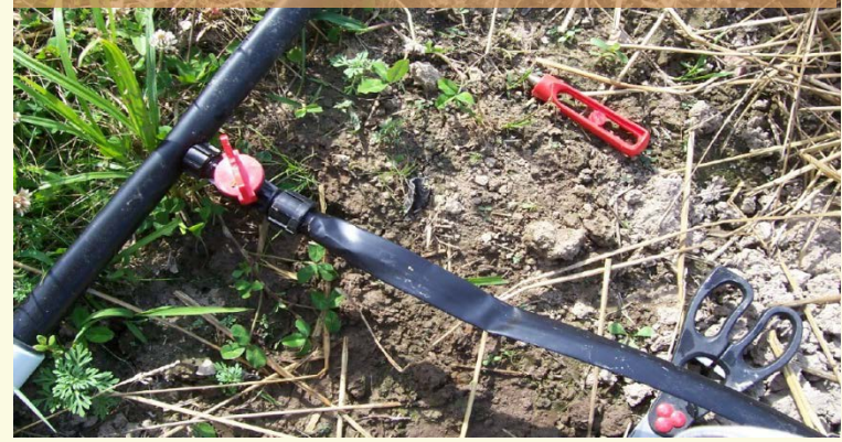
Push tape on & tighten collar nut
