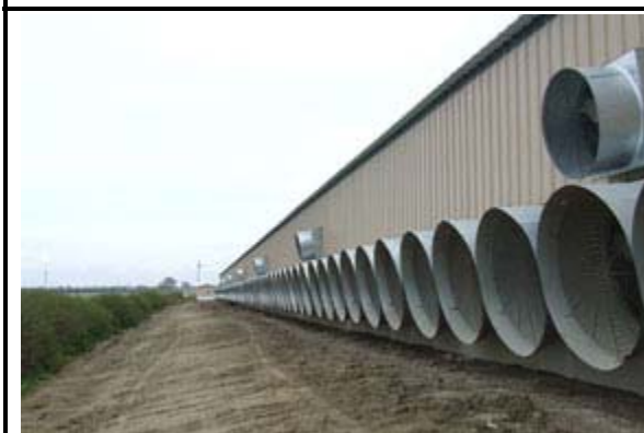
Mechanical Ventilation Freestall Barn
