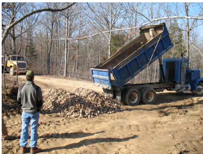
To avoid a poor situation later, anticipate wet soil conditions and have road rock delivered prior to hauling logs.
