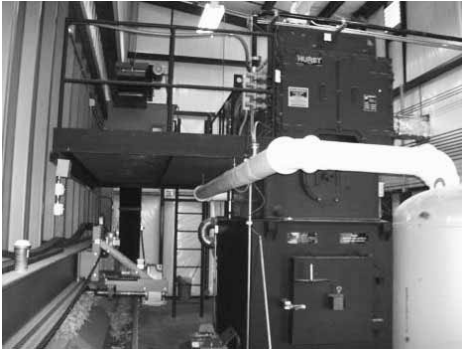
Wood chips are augured from a storage bin onto a conveyor (lower left) to the combustor which sits beneath the boiler (right).
