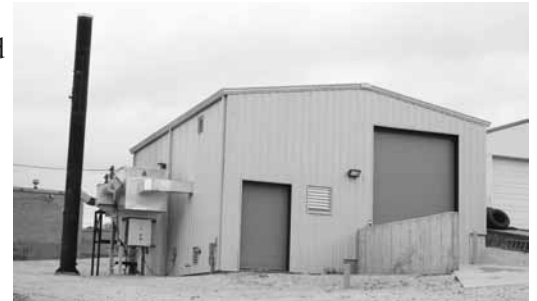
Ellington Fuels for Schools project. All projects are equipped with electrostatic precipitators (unit between building and smoke stack) to reduce particulate matter.
