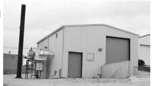
Ellington Fuels for Schools project. All projects are equipped with electrostatic precipitators (unit between building and smoke stack) to reduce particulate matter.
