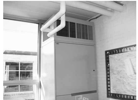
Heat exchangers like this one at Gainesville help to distribute heat evenly throughout the school.
