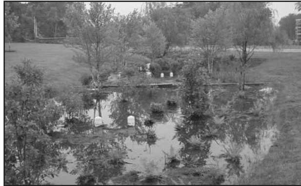
Bioretention basins are designed to absorb runoff from impervious surfaces such as roadways and parking lots.
